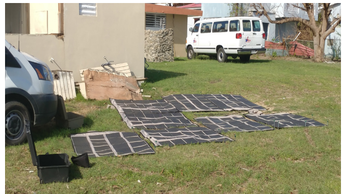
Figure 6 - Solar Stik System Deployed
