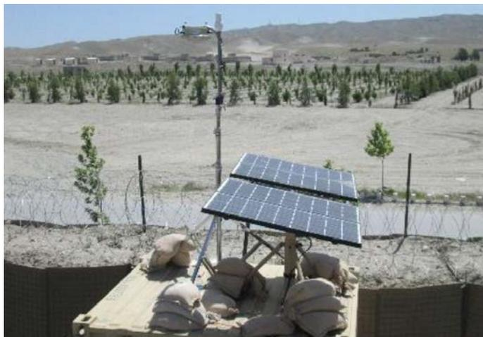
Figure 7 - Solar Stik System powering RFID Interrogator at a convoy rest stop
